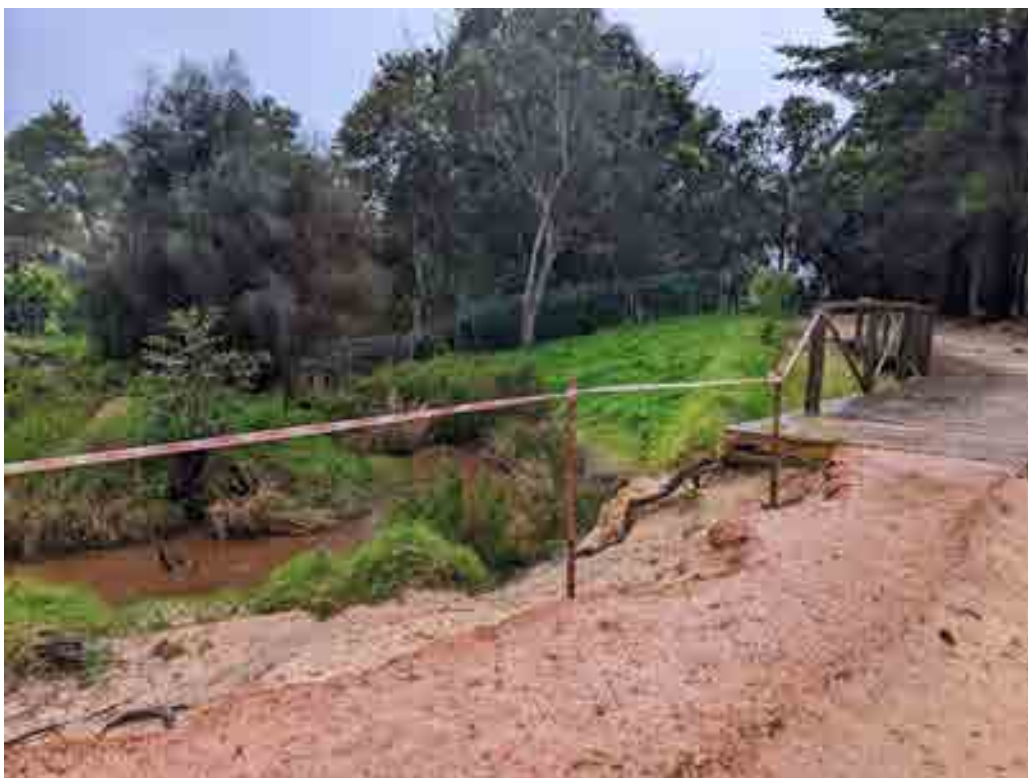
Figure 10b: the erosion (exacerbated by user activity) is clearly visible at the end of the boardwalk.
