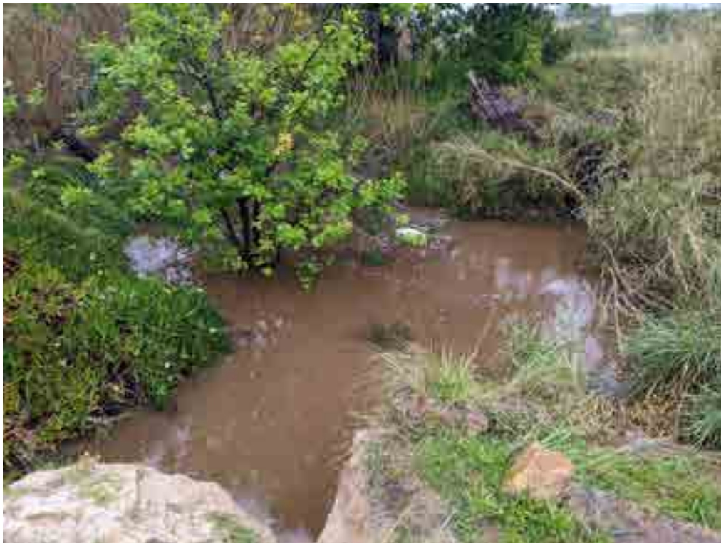
Figure 9: Erosion and widening of the river below the gabions at the Labrador Pool. The bank in the foreground is in a constant state of erosion.
